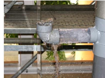
Photo 2: Spouting of water from backflow pipe
