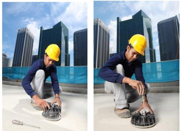
*Siphonic System - Pipes and outlets installation*
