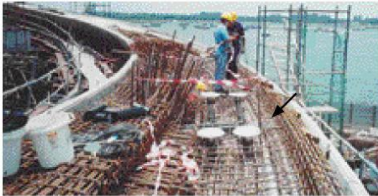
Siphonic outlets installation at the lowest section of the sloping gutter.
